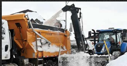
Truck Loading Chute
